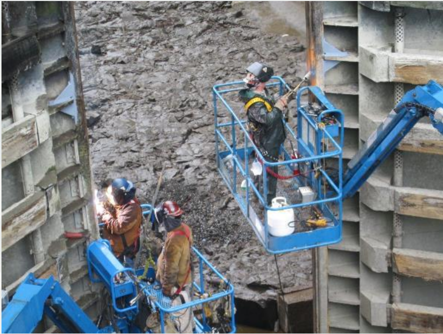
2017 McNary Downstream Gate weld repairs
